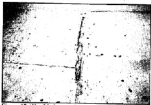
Figure 10: We did observe this 27 inch by 2 inch seam crack. It is less than 1/4 inch deep, thus not much of a hazard.
