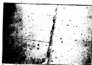
Figure 11: Another seam crack 8 feet long, but again, not very deep is located nearest the public sidewalk.
